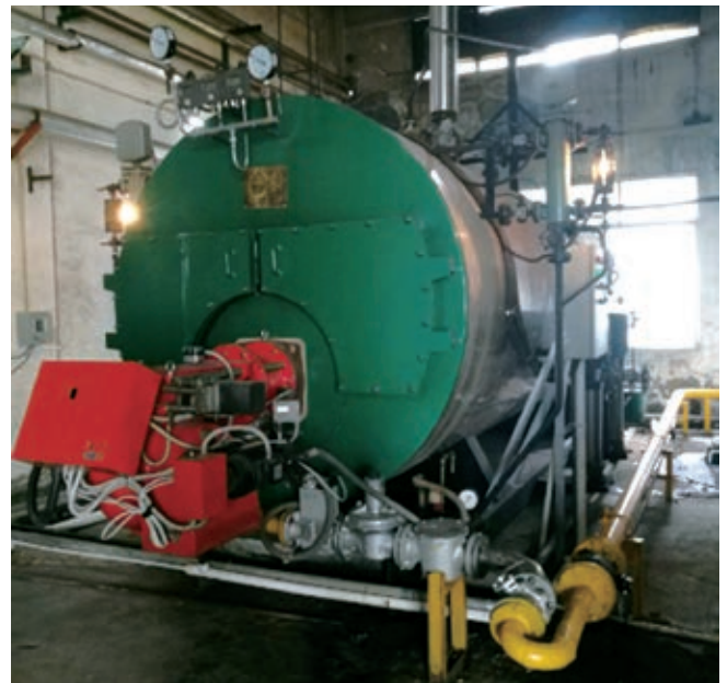
The natural gas boiler in Zhongshan Tungtex
