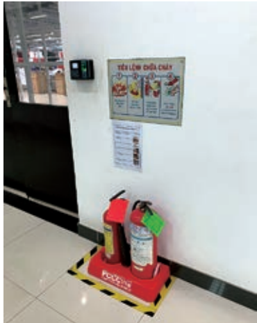
Fire extinguishers and fire slogans are placed in the factory
