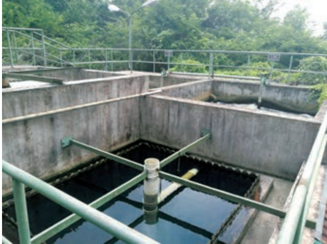
The sewage treatment facilities in Zhongshan Tungtex
