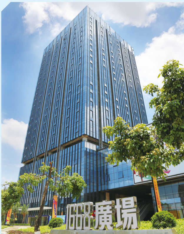
Office tower of 1668 Square in CSC Nanning 於南寧華南城1668廣場寫字樓
