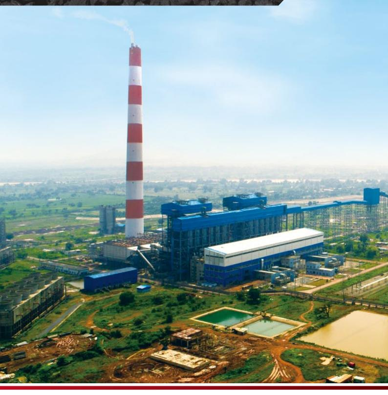
Agritrade Resources's energy business engaged in the operation of a high powered domestic coal based thermal power plant comprising of four units of 300 megawatt each, in two phases of 600 megawatt each, at village Binjkote & Durramuda, Raigarh, in the State of Chhattisgarh, India.
