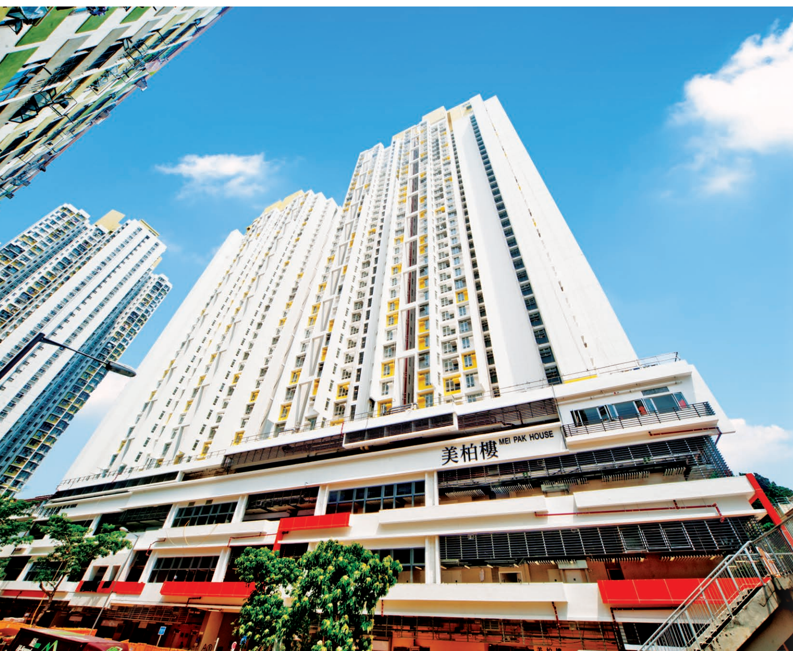
Public Housing Project at Shek Kip Mei Estate Phase 6
