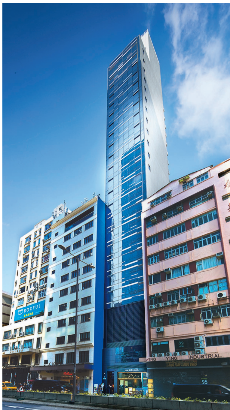
The commercial building in Kwun Tong
