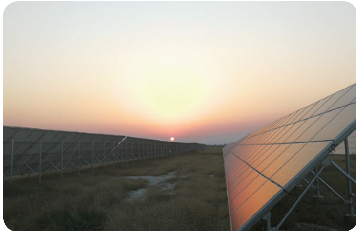
Kezuo Zhongqi Solar Project
