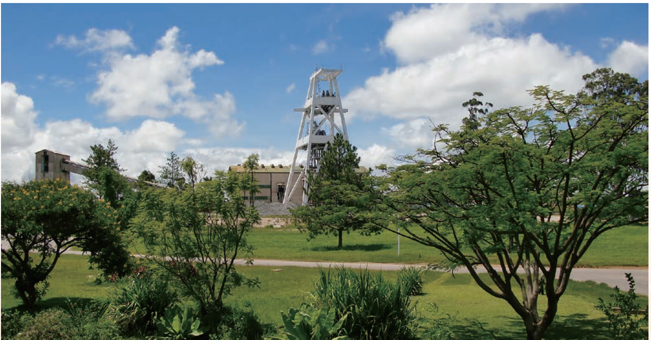
Central auxiliary shaft of Chambishi West Mine
