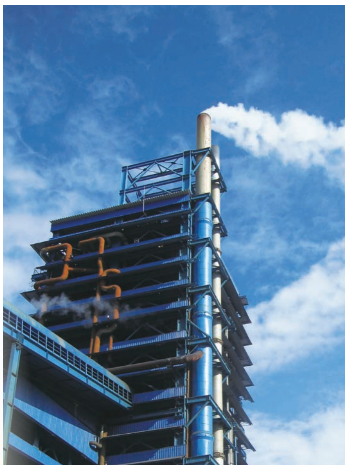
ISA furnace of copper smelting company
