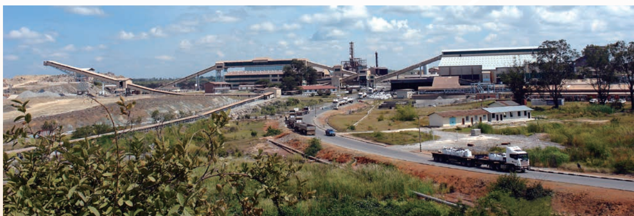
Panorama of the ore processing plant of Chambishi Copper Mine
