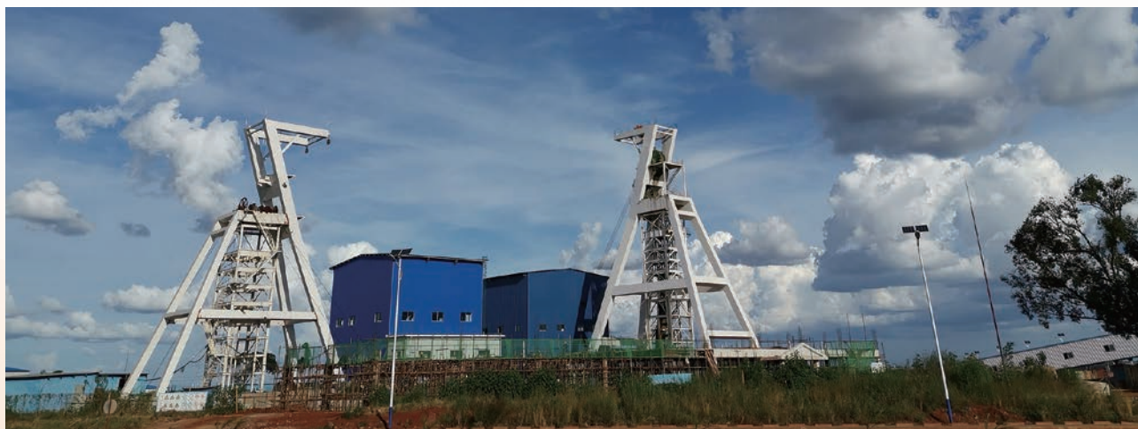
The main shaft and auxiliary shaft of Chambishi Southeast Mine
