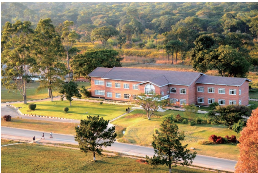
NICA office area
