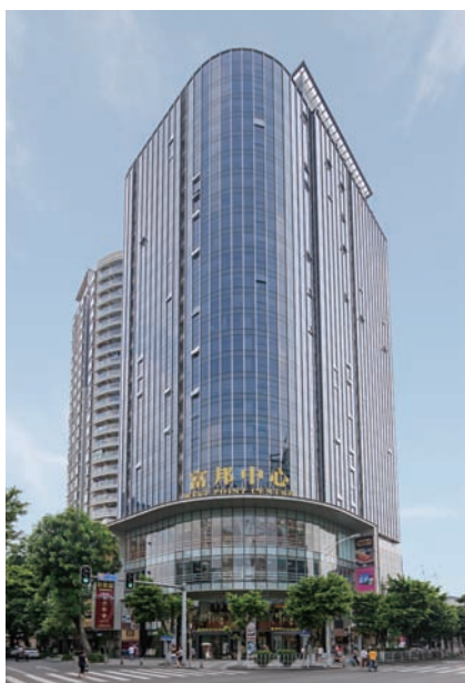
Guangzhou West Point
