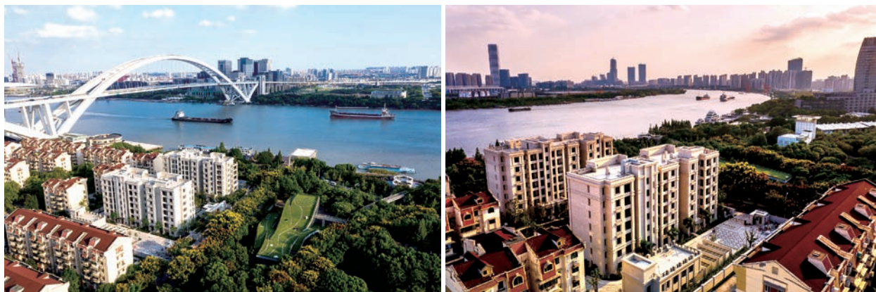
Shanghai Wuli Bridge Project
