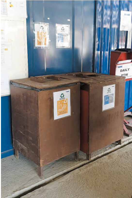
Recycling station in the worksite of Bangsar 61, Kuala Lumpur.
