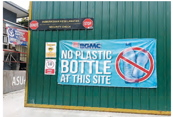
"No Plastic Bottle" banner at the entrance of worksite at Bangsar 61, Kuala Lumpur.
