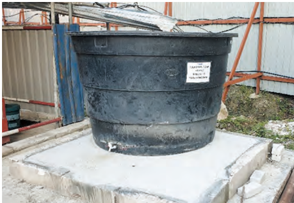
Rainwater harvesting system installed at the worksite of Bangsar 61, Kuala Lumpur.
