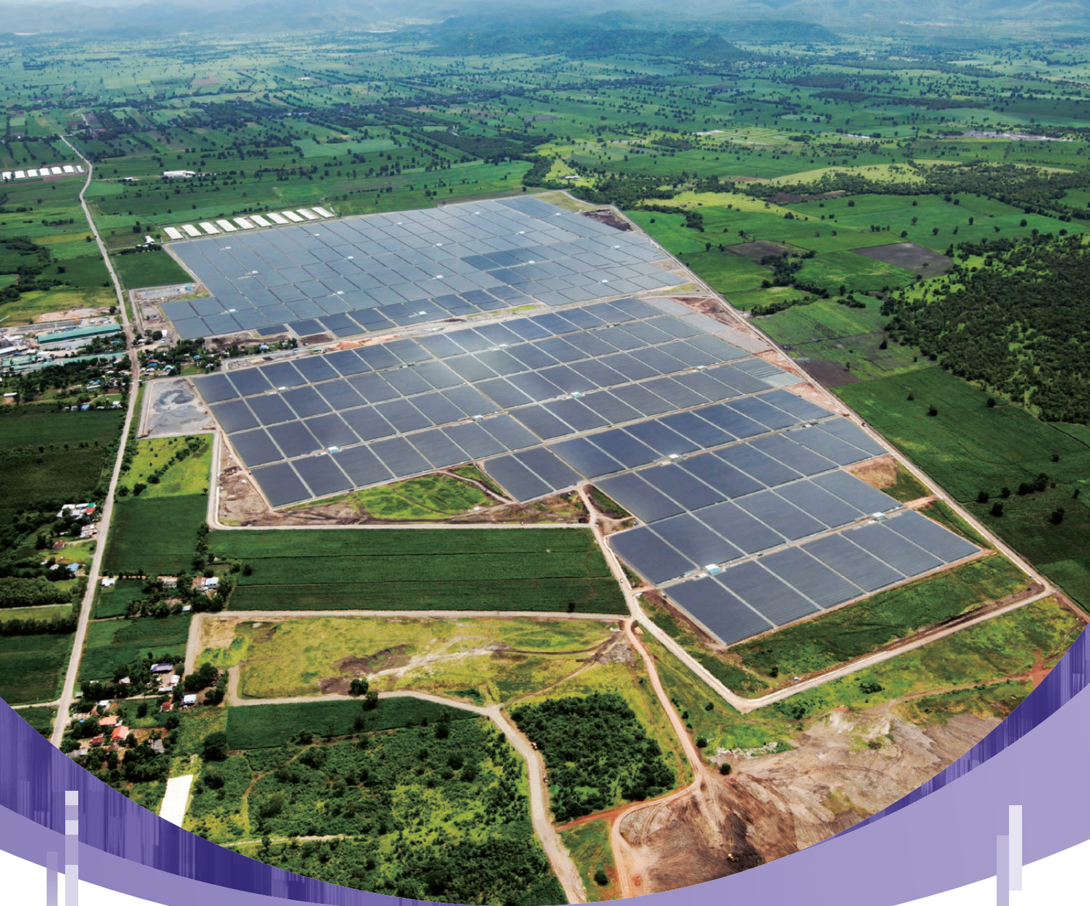
Lopburi Solar Farm
