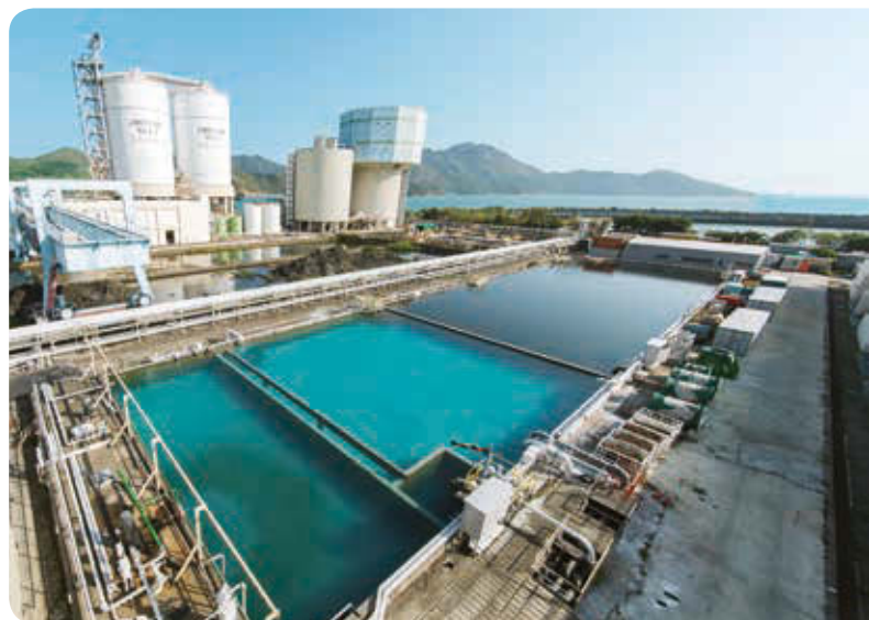
▲ Rainwater and plant processing water are collected at Lamma Power Station for reuse and help cut down on fresh water used.
