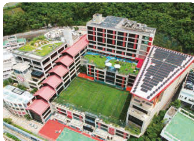
▲ Canadian International School has joined HK Electric's Feed-in Tariff Scheme and installed large-scale solar power system in the campus.
