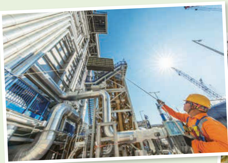
▲ Selective Catalytic Reduction System under installation.
