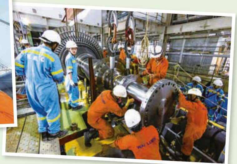
▲ Engineers are assembling steam turbine for L10 generating unit.
