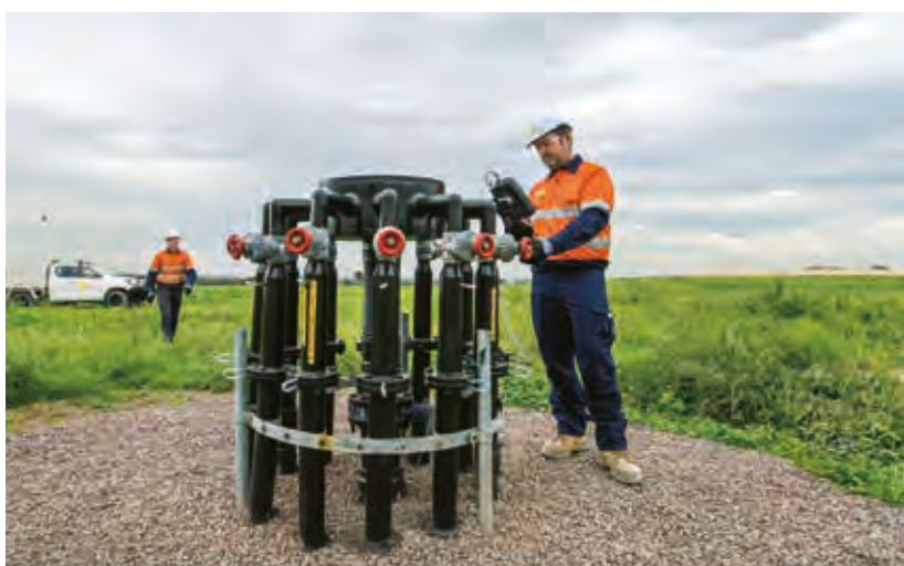
Technicians calibrating a gas well at EDL’s Lucas Heights power station in New South Wales. EDL has led the way for the landfill gas generation sector in Australia for decades.
