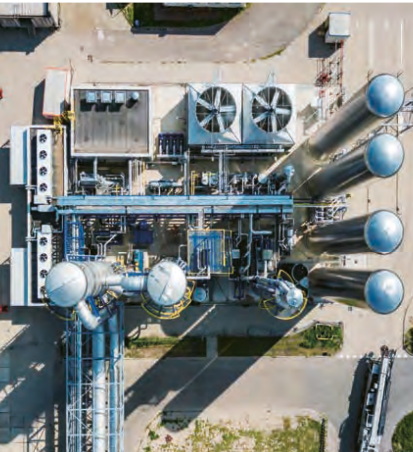
AVR’s pioneering CO 2 capture and liquefaction setup allows carbon emissions to be reused for greenhouse cultivation.
