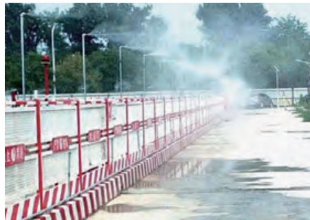
Example of using water sprinkler system to prevent dust from airborne.
