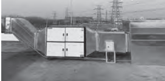
汰換老舊排油煙設備 Replacement of out-dated fume exhaust equipments
