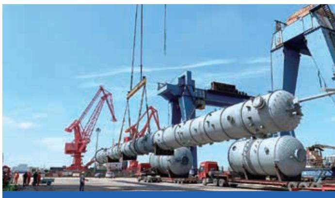
The three reactors were stirred tank reactors of 110 tons each. The pyrolysis gas gas phase dryers weighed 250 tons each, with special structures which required exceptional technics.
