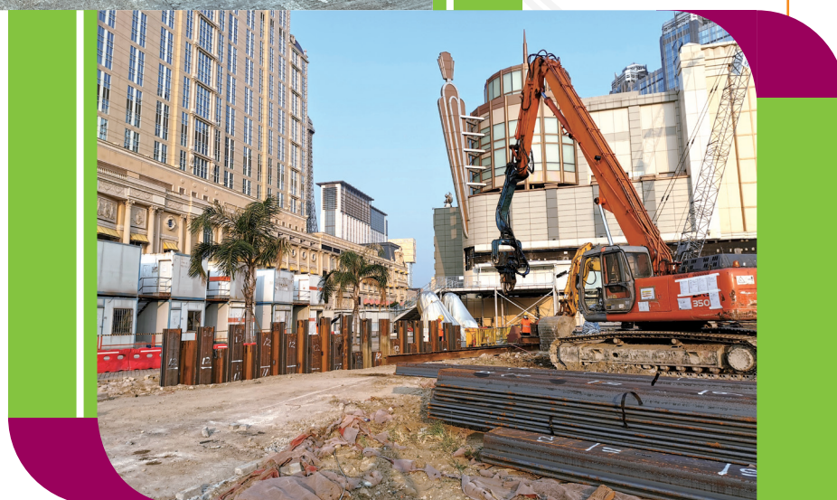
Sheet piling works for a new hotel complex at Cotai, Macau
