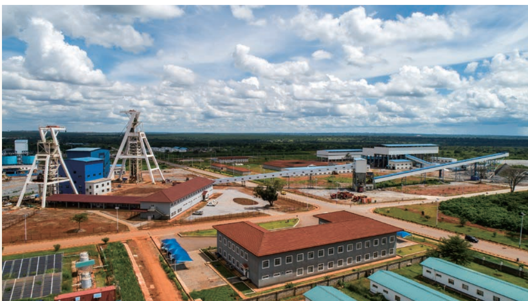
Production and Control Centre of NFCA Southeast Mine
