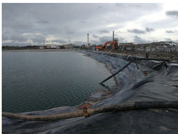
Utilisation of tailings pond backwater
