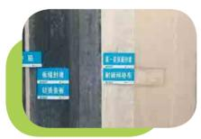
Construction method for interior wall: hollowing and cracks are effectively controlled by using lightweight panels of autoclaved ceramsite concrete for partition wall.
