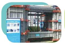
Construction method for aluminum mold: achieve accurate control of vertical deviation of wall column and ceiling level difference within 5mm in 11 processes.
