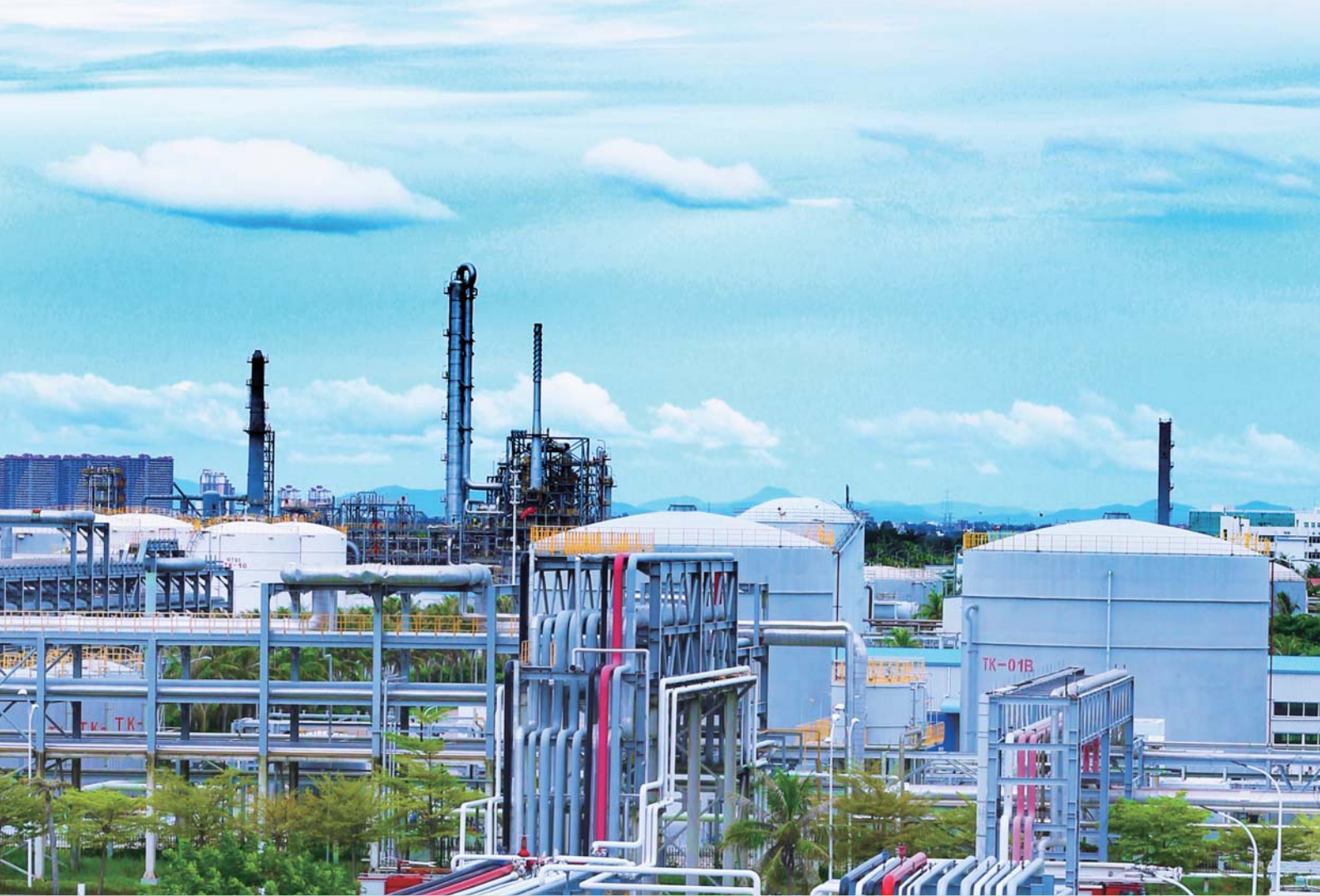
Oil and gas pipeline of Hainan area two
