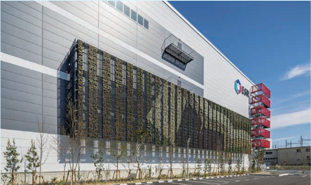
ESR Ichikawa Distribution Centre, Japan features an impressive “green wall” that acts as a sound-proofing barrier and helps to reduce urban heat-island effect while cleaning the air of pollutants and dust.
