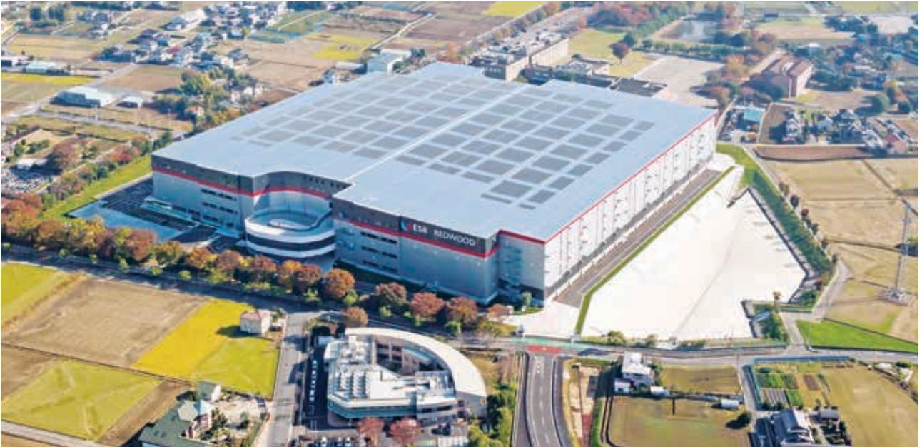
ESR Kuki Distribution Centre in Tokyo is a four-storey state-of-the-art facility with roof top solar panels providing 2.3MW of clean energy installed capacity. It has been certified as a Class A property under CASBEE—Japan's national building sustainability rating system.
