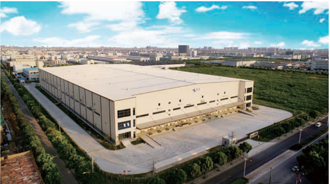
Shanghai Fengyuan Logistics Centre, China
