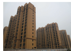
Xingwei Resettlement House Phase I
