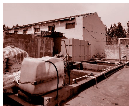
Sewage treatment station
