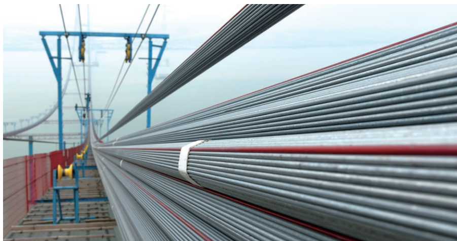
Construction site for cable installation
