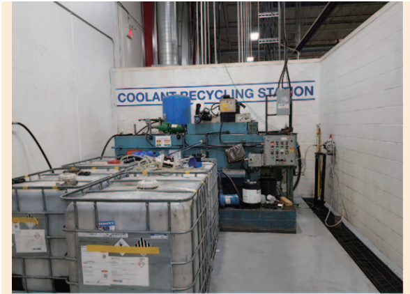
In Ancaster, Canada, the site reviewed its onsite coolant recycling programme and determined that it could reclaim more coolant, saving of 38,000 litres of coolant concentrate and 450,000 litres of water a year
