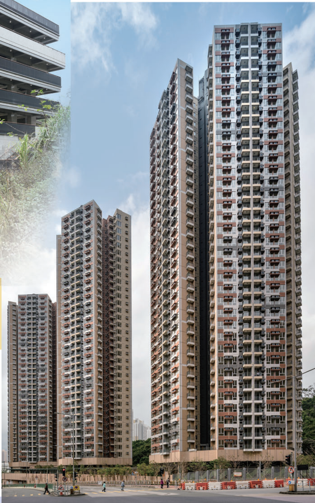
Main Contract for Subsidised Sale Flats Project at Shatin Area 36C 沙田36C區地皮發展資助出售房屋項目總合約
