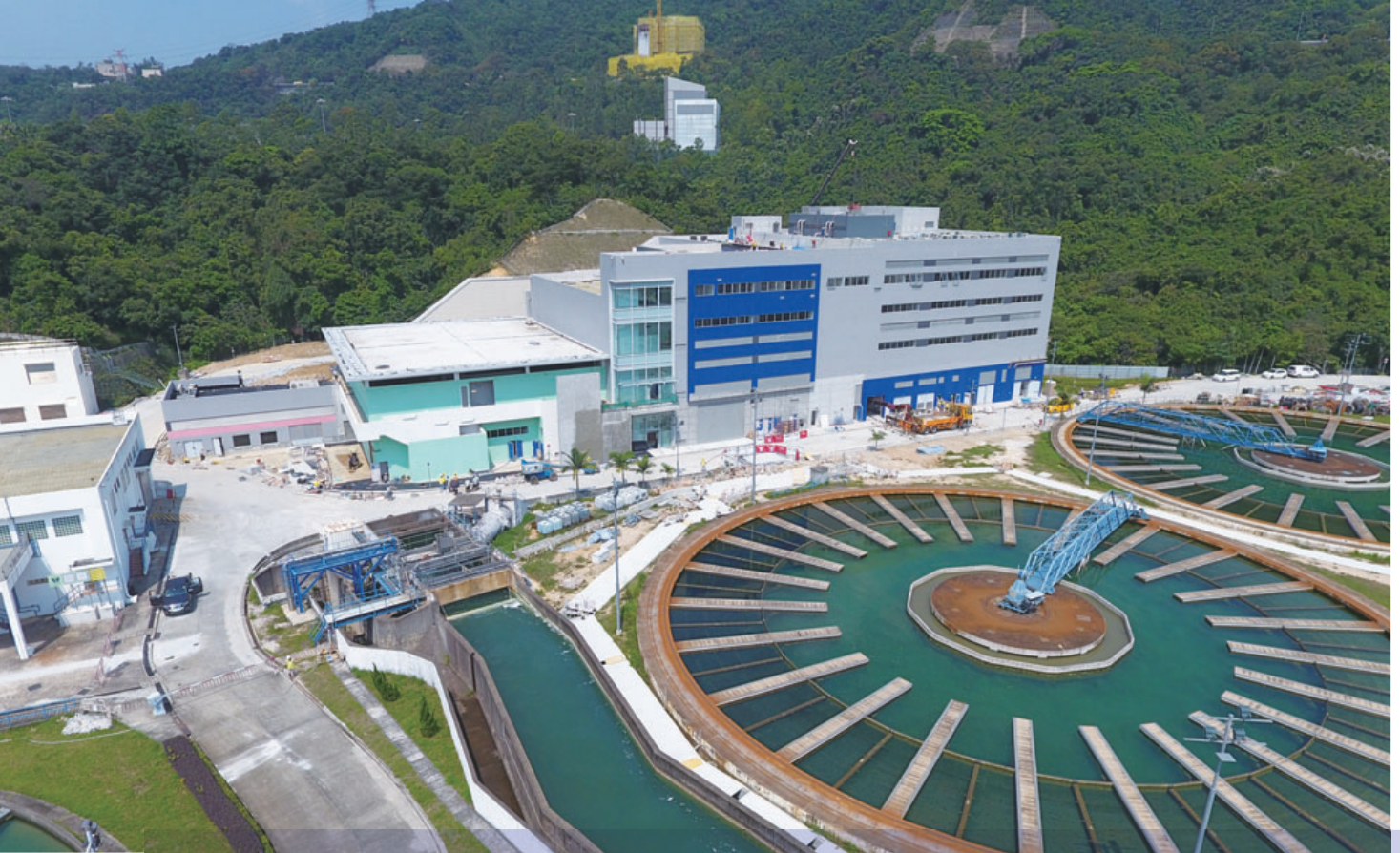
In-situ Reprovisioning of Shatin Water Treatment Works (South Works) — Advance Works 沙田濾水廠原地重置工程 (南廠) — 前期工程
