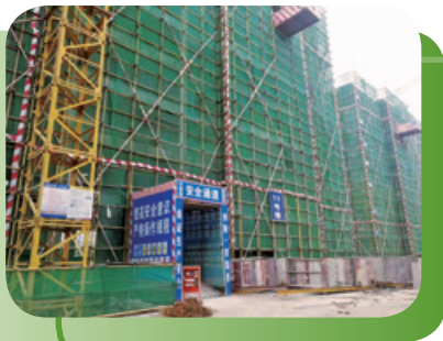
Safe passageway at the construction site 施工現場安全通道
