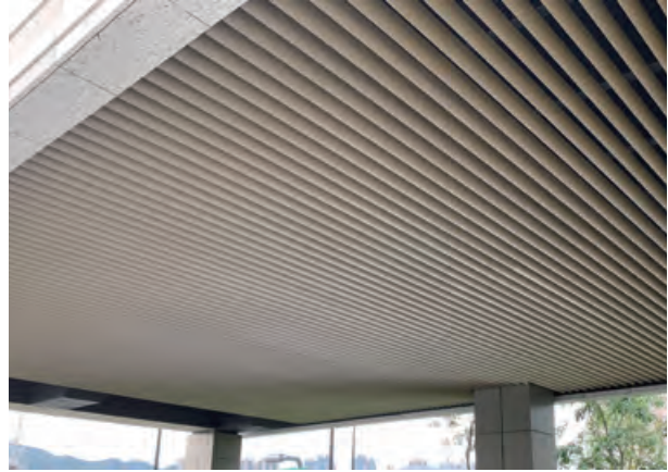
Supply and installation of suspended ceiling system for Lohas Park Package 7A & B 日出康城第7A及7B期 – 供應及安裝假天花系統
