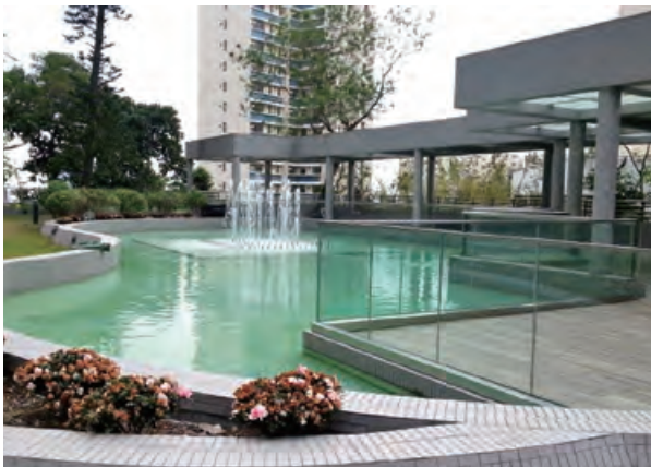
Building renovation works of Cavendish Heights (Block 1-7) at 33 Perkins Road, Jardine's Lookout 渣甸山白建時道33號嘉雲臺(1-7座)樓宇之裝修工程
