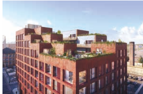
Roof Terraces, New Cross Central, Manchester
