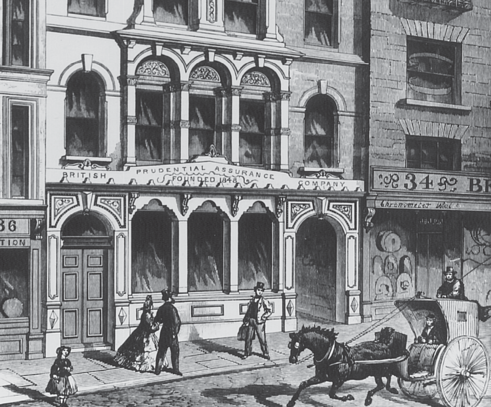
Prudential's office at Ludgate Hill, London; from The Building News , 1863.
