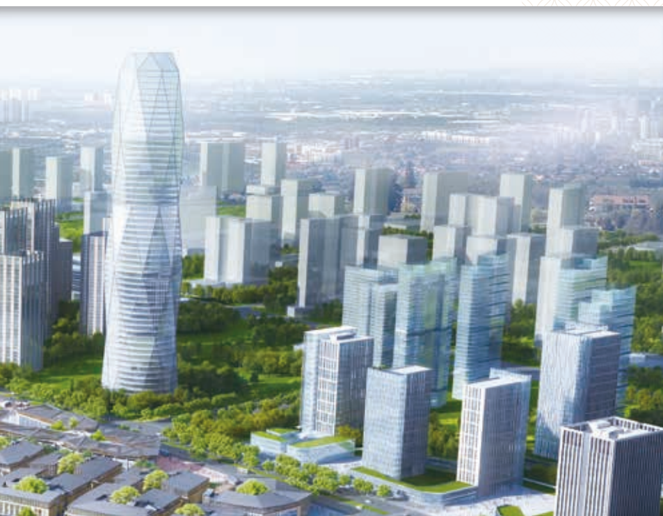
Beijing Canal Financial Headquarters
