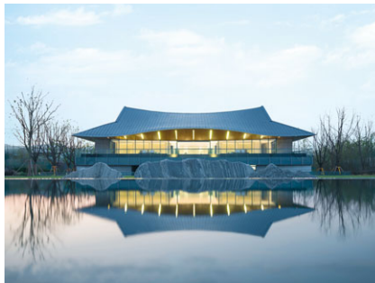
蘇州吳中區西山項目 Suzhou Wuzhong District West Mountain Project
