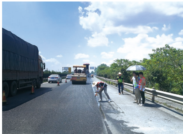
Test-trialling bituminous mix with used tyre materials for road maintenance
