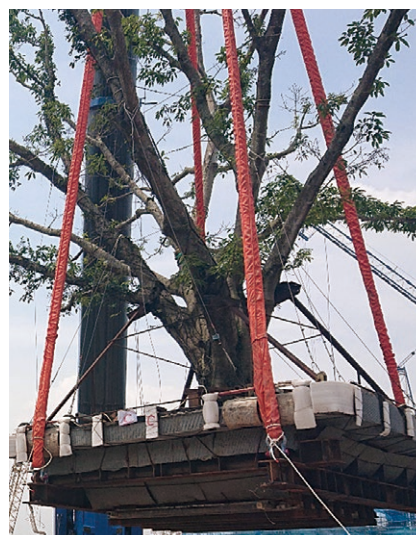
Tree conservation through transplanting at a Public Housing Project in Queen’s Hill, Fanling
