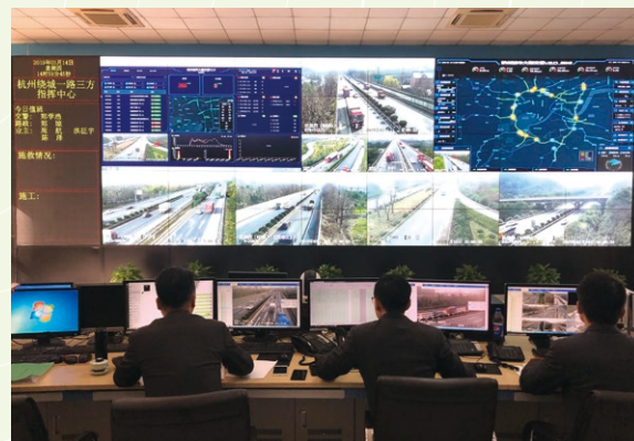
Real-time automated monitoring, intelligent dispatch and vehicle management
