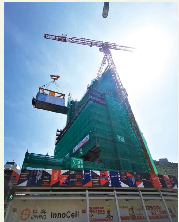
Constructional phase of InnoCell at Hong Kong Science Park
