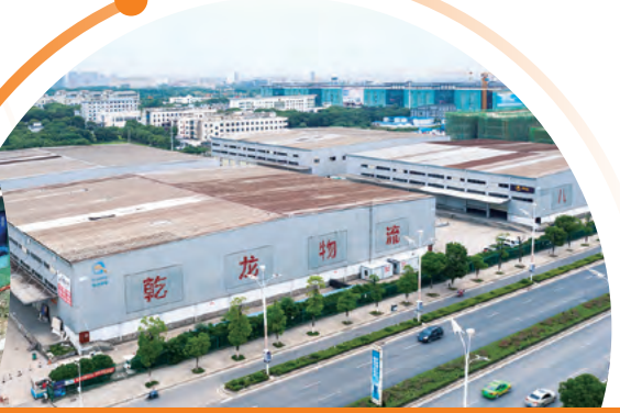
Qianlong Logistics Park in CSC Nanchang 於南昌華南城的乾龍物流園
