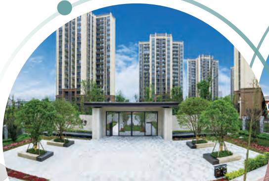
Residential ancillary in CSC Chongqing 於重慶華南城的住宅配套
