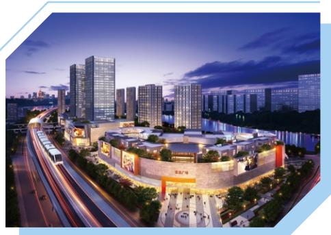
HANGZHOU QINGSHAN LAKE POWERLONG PLAZA PHASE I
