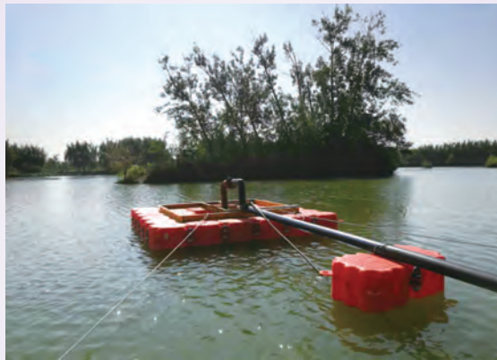
Jiangsu Texhong: “Texhong Lake” water-drawing renovation 江蘇天虹：「天虹湖」取水改造
