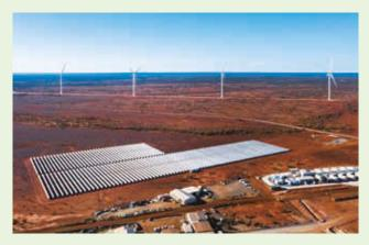
EDL's Agnew hybrid renewable project is Australia's largest renewable microgrid and a test bed for innovative hybrid energy generation. The 56-MW microsite, located at the Gold Fields Agnew gold mine, incorporates a mixture of wind, solar and thermal generation and battery storage.
