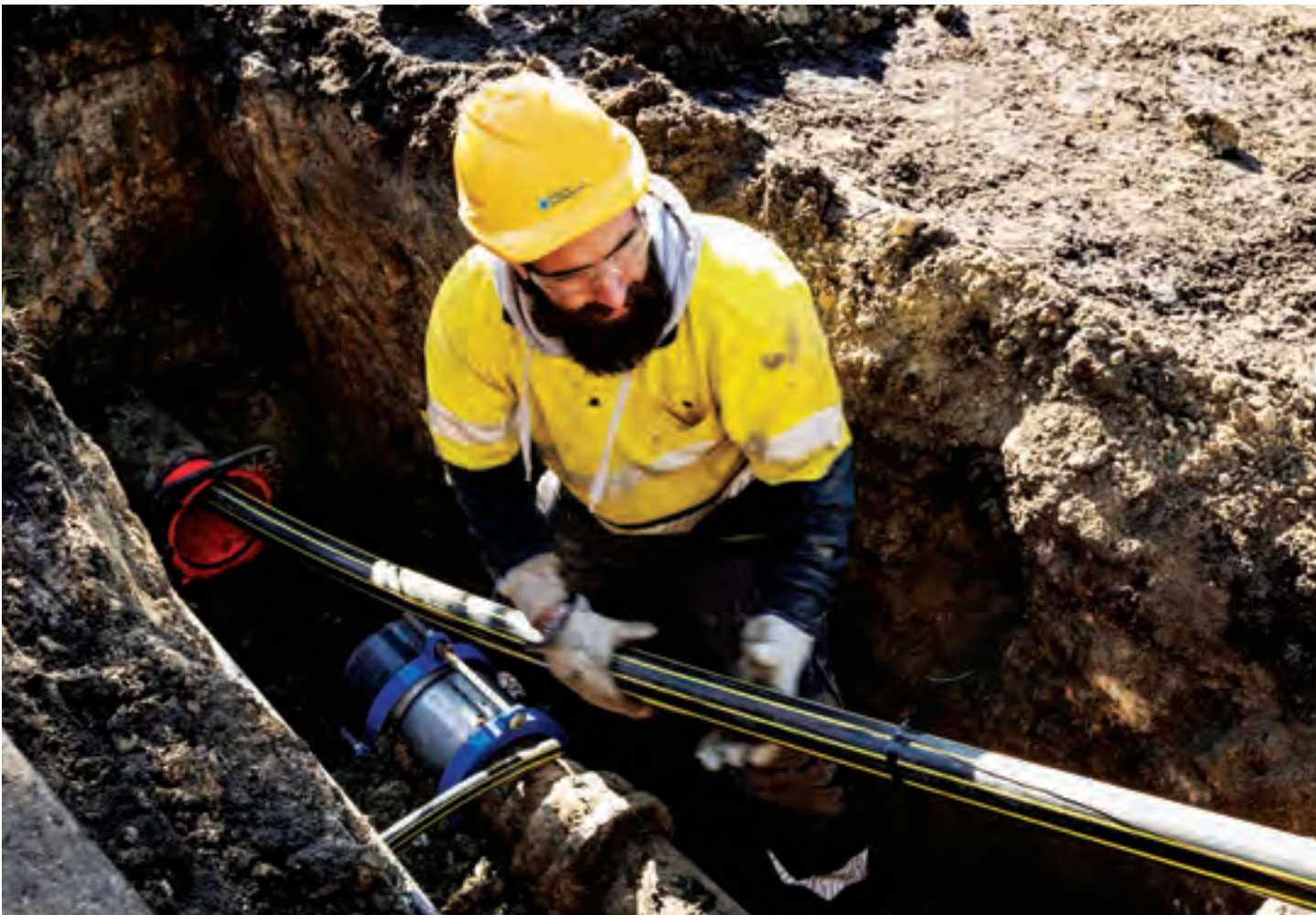
Multinet Gas completed the replacement of 133 kilometres of old cast iron mains ahead of schedule.
