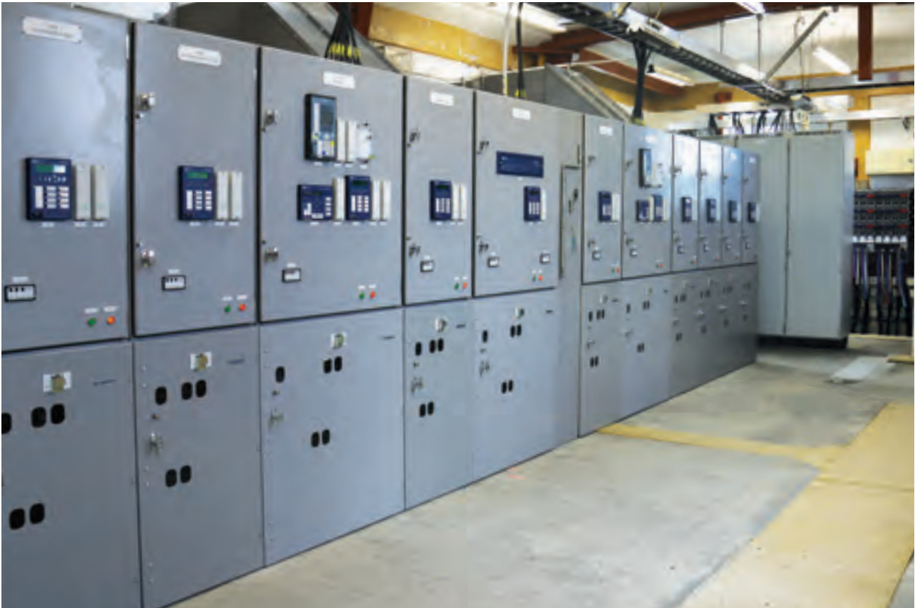
Wellington Electricity's three-year Earthquake Readiness Programme, which aims to reduce outage times following major earthquakes, is near completion.
