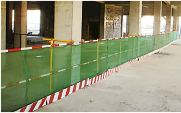
Stairs and balconies edges are equipped with protective facilities such as stable railings to protect workers' construction safety.
