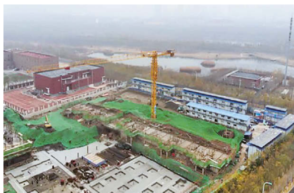
Example of covering up of construction area.
