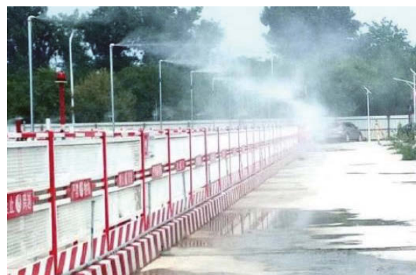
Example of using water sprinkler system to prevent dust dispersion.
