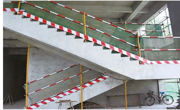
Stairs and balconies edges are equipped with protective facilities such as stable railings to protect workers' construction safety.
