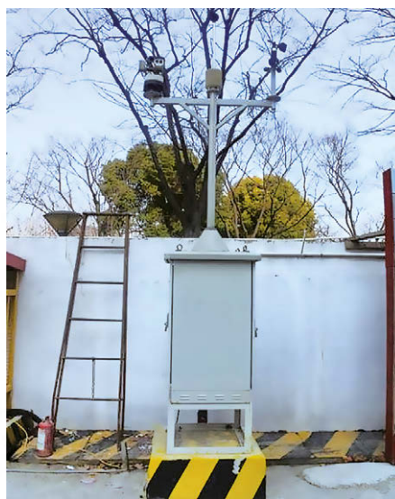
Noise dosimeters are installed at construction site to monitor noise level. Meter reading is recorded few times a day at random intervals serving as random inspections.
