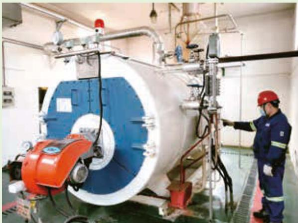
The chemical company of the oilfield chemical division changed the boiler fuel from diesel to alcohol-based fuel, reducing diesel consumption by 85 tonnes per year and carbon dioxide emissions by 264.77 tonnes
