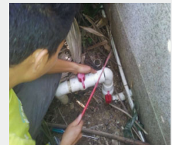
Routine maintenance of water supply equipment
