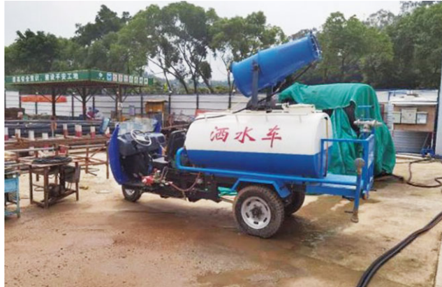
Sprinkling and dust control equipment on the construction site
