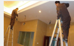
Switch circuit retrofit
