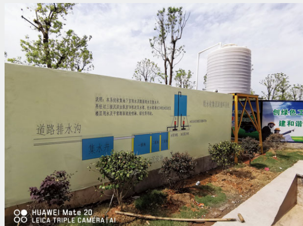
Rainwater collection system on construction site
