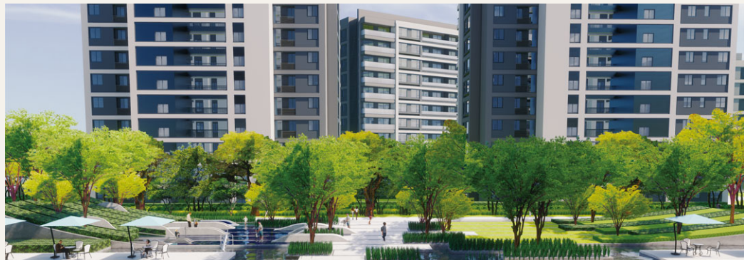
Measures for storing rainwater and adjusting the rainwater discharge rate through ecological environment
