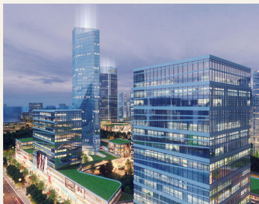
Business view of Shijiazhuang HOPSCA Center (石家莊融創中心)
