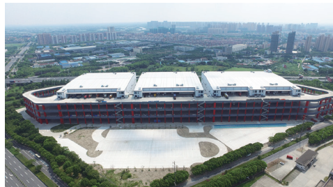
江蘇崑山易商物流園 Jiangsu Kunshan E-commerce Logistics Park
