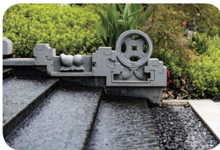
Staircase with festoon sculpted head (垂帶雕飾狀收頭) in Jianfa & Jiulongcang • Yangxi* (建發&九龍倉•央璽) Project of Guangzhou
