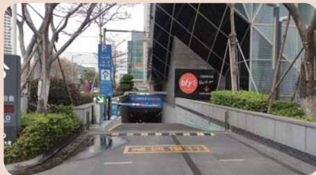
Actual view of a smart car park
