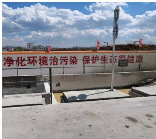
Sewage tertiary sedimentation tank 污水三級沉澱池
