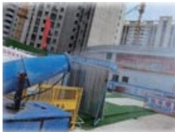
Mist cannons at the entrance and exit of construction sites
