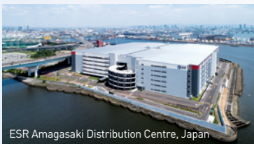
ESR Amagasaki Distribution Centre, Japan
