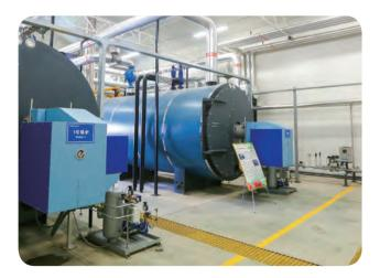
By setting up hot water storage system and carbon dioxide recycling system for the greenhouse production base, while the natural gas boilers are heating up the greenhouse with combustion of natural gas, the carbon dioxide generated would be supplied to the greenhouse crops for photosynthesis. Crop yields would be increased and zero emission of carbon dioxide from natural gas boilers would be achieved.
