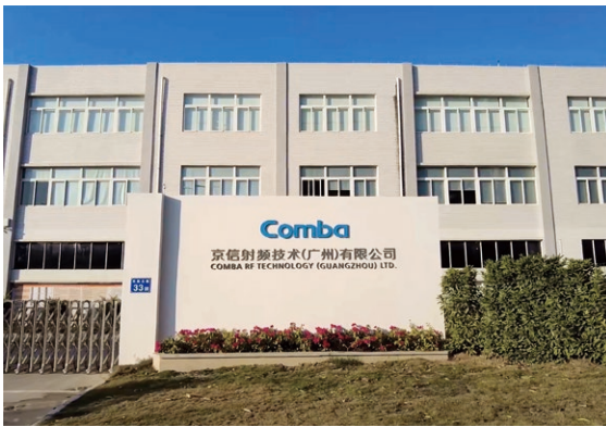
The 5G antenna and filter production base in Zhongxin Guangzhou Knowledge City commenced operation
