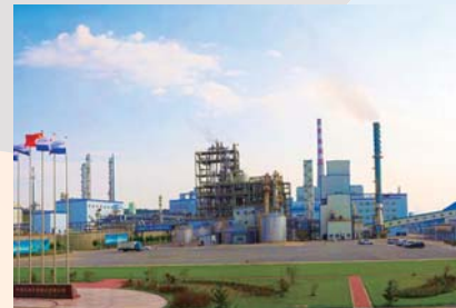
The production facilities in Heilongjiang
