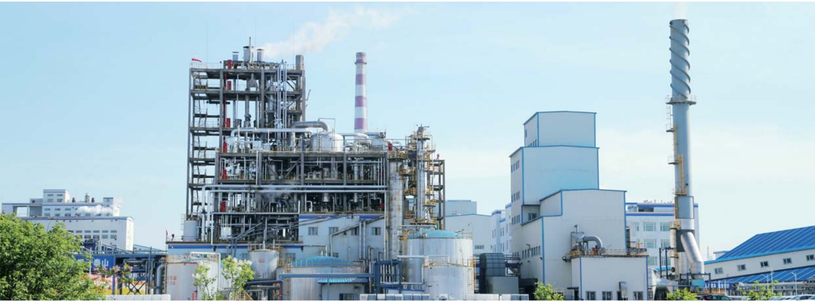
■ CNOOC Huahe urea plant
