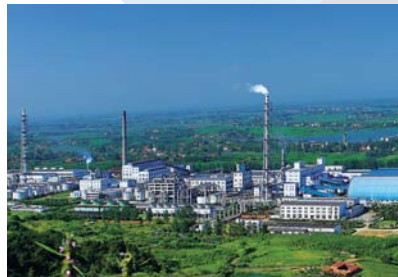
The production facilities in Hubei
