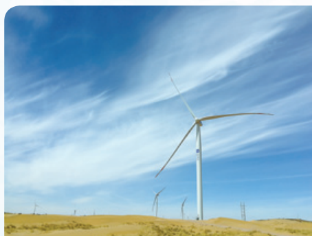
Wind Power Plant, Alashan, The Inner Mongolia Autonomous Region
