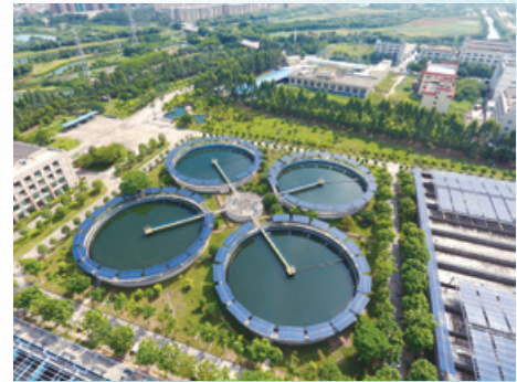
Distributed Photovoltaic Power Plant in a water plant of BEWG, Dongguan, Guangdong Province
